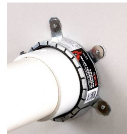
Plastic pipe (firestop collar)
