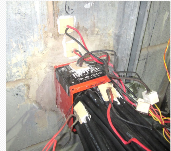
Thermocouples to measure temperature
