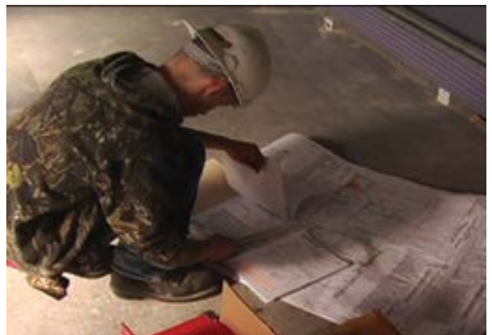
Fire-resistance inventory includes life safety drawings, manufacturers' instructions, listings, and safety data sheets. FCIA Photo
