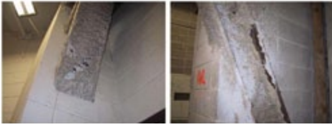
SFRM's Maintenance Patching is required for continuous fire-resistance maintenance. GCP Applied Technologies, Inc. Photo
