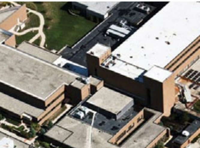
Roof Coverings matter when part of the fire-resistance rated assembly. Waukegan Roofing Photo
