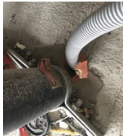
Even when warning stickers exist, (on pipe), services breach firestops. Pro-Firestop Photo
