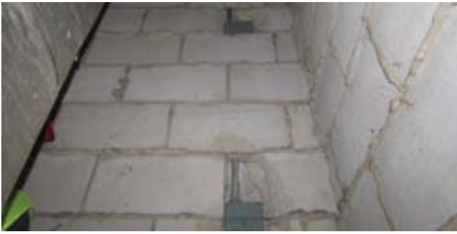
Concrete block assemblies for walls, shafts, can be found listed in the U900 series designs in the UL Product iQ Database. C. Zussman, Pepper Constr. Photo.
