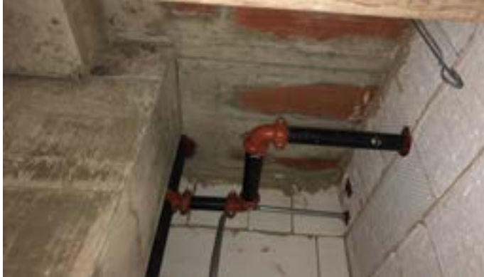
Gypsum Block Assembly, with firestopping. C. Zussman, Pepper Constr. Photo
