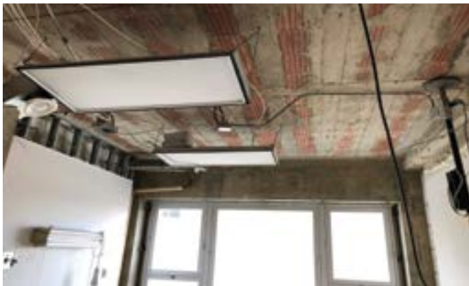
Clay tile and concrete horizontal assembly. C. Zussman, Pepper Constr. Photo
