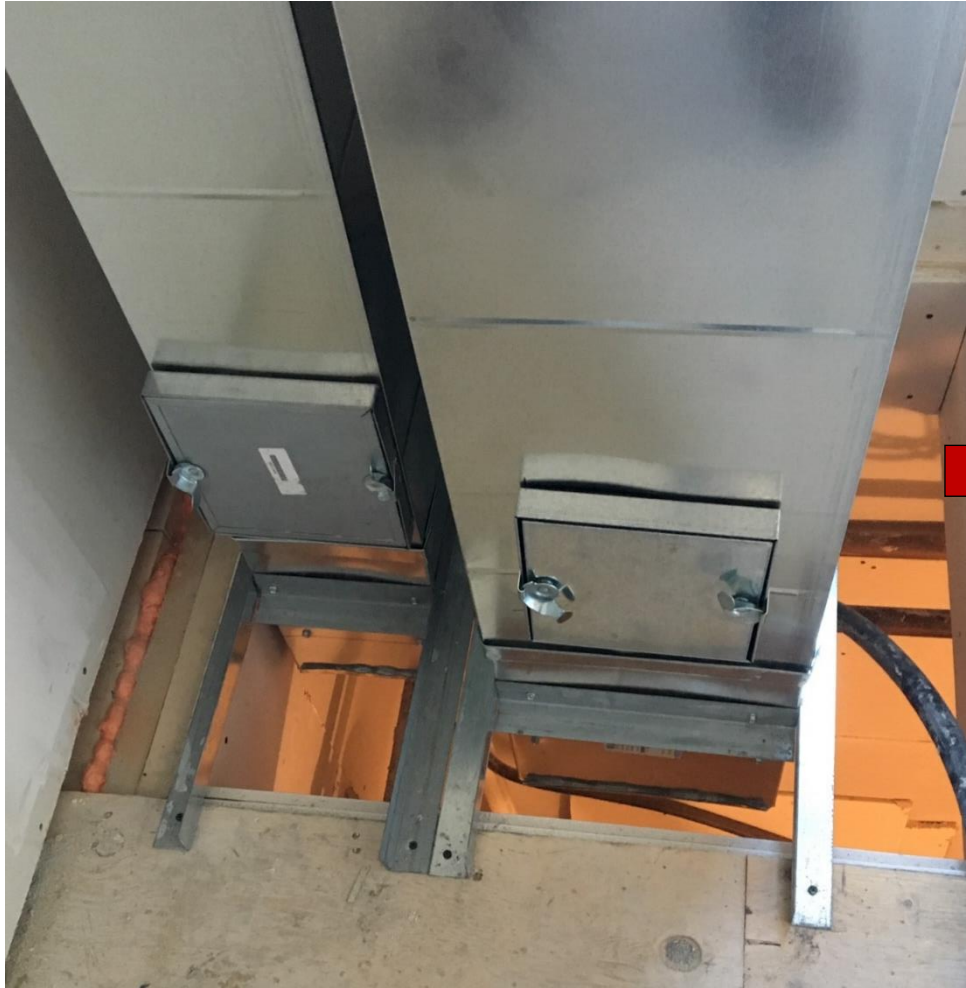
Fire Damper Annular Space?
