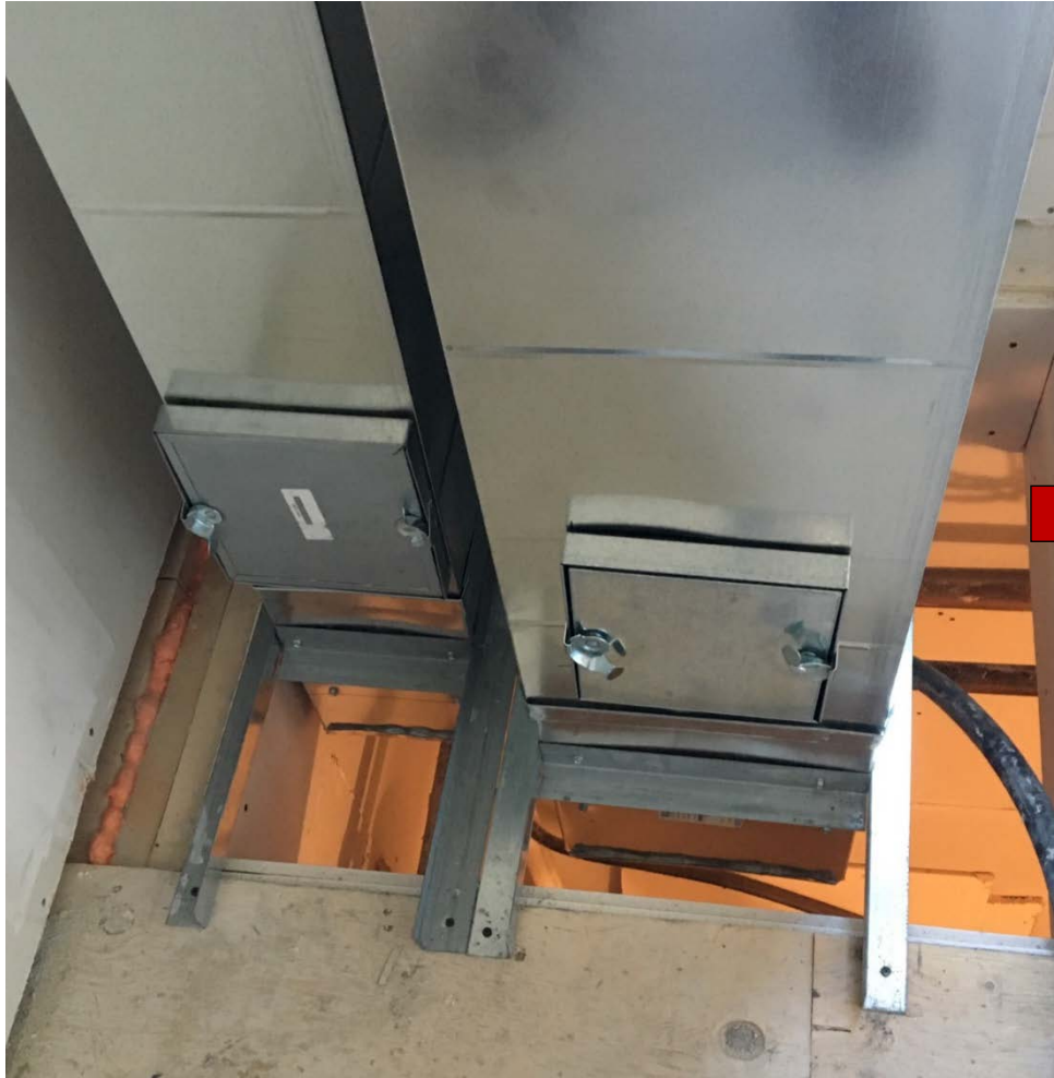
Fire Damper Annular Space?
