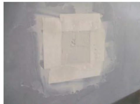
Figure 5: Tape and Finish Patched Area
