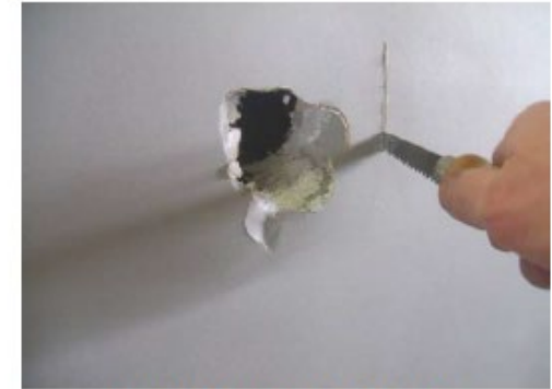
Figure 2: Square Off Damaged Area
