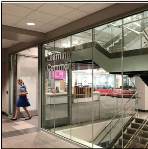
Fire-resistance-rated Wall
