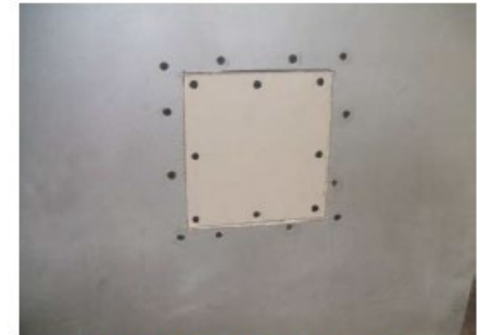
Figure 4: Apply Gypsum Panel Patch
