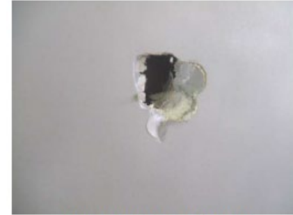
Figure 1: Damaged Gypsum Panel
