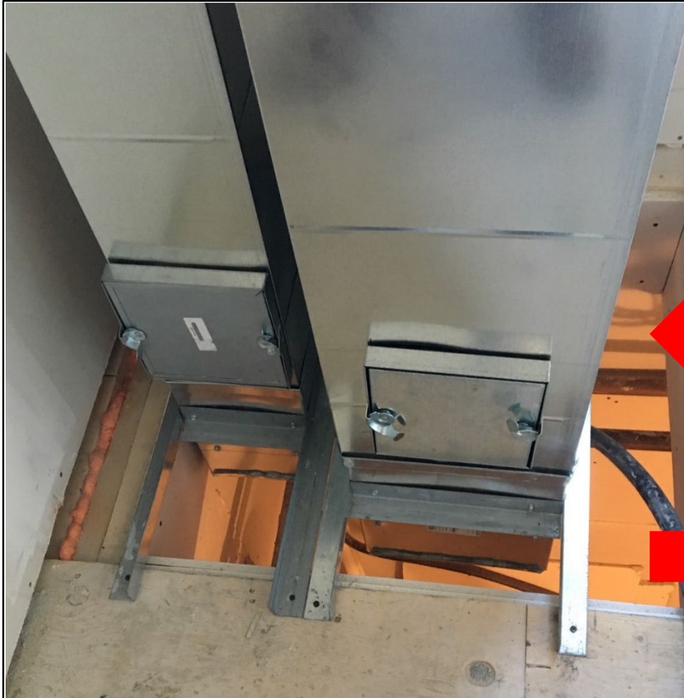
Fire Damper Annular Space?
