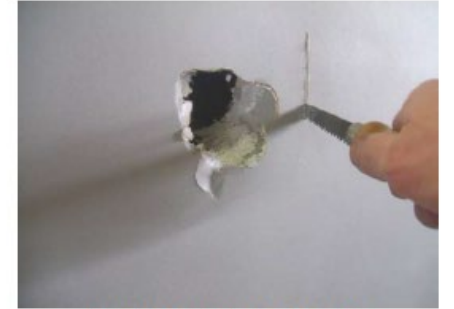
Figure 2: Square Off Damaged Area
