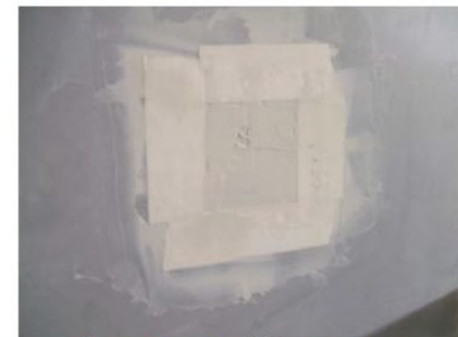
Figure 5: Tape and Finish Patched Area
