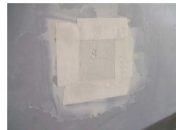
Figure 5: Tape and Finish Patched Area
