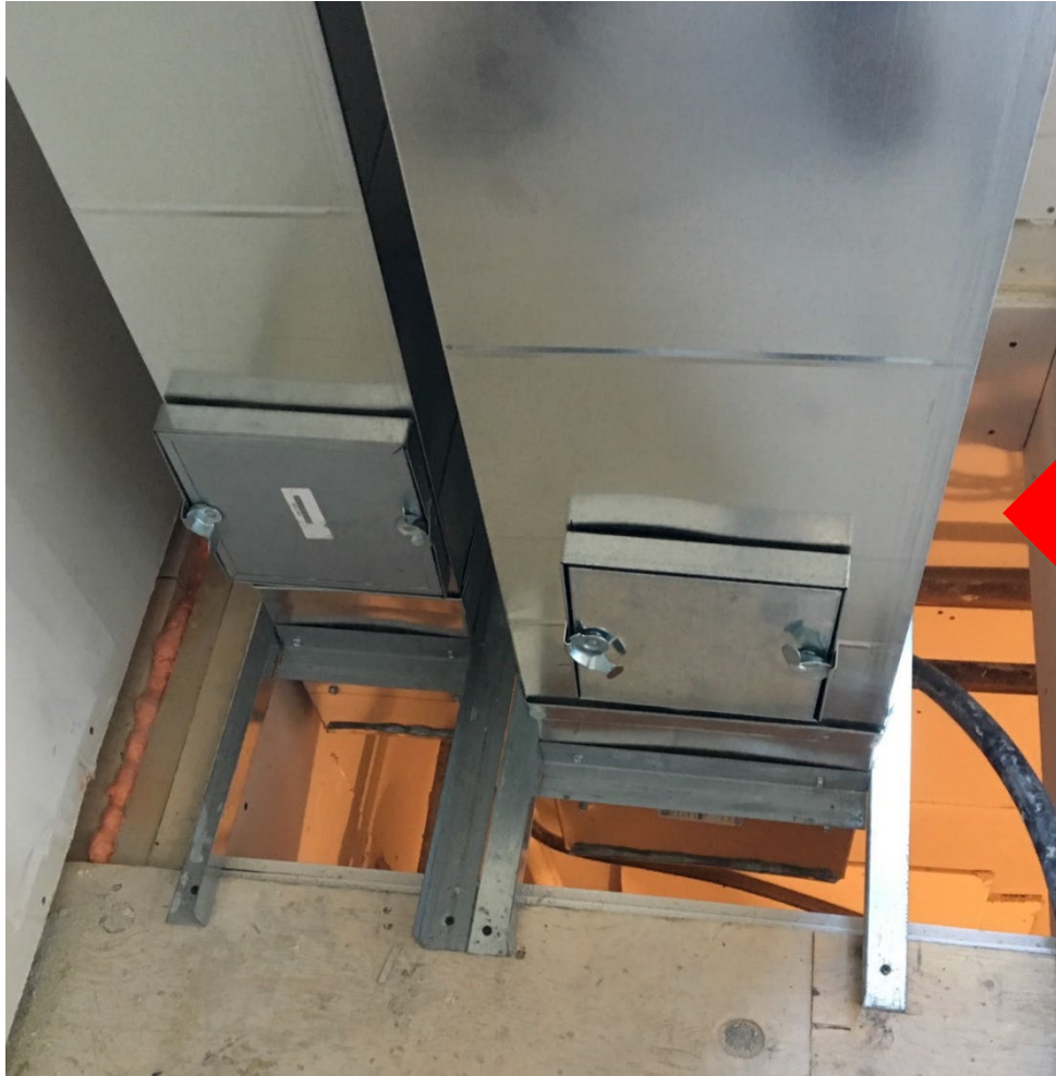
Fire Damper Annular Space?
