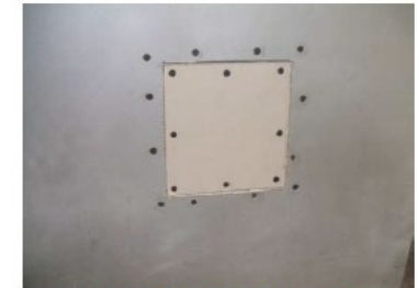
Figure 4: Apply Gypsum Panel Patch
