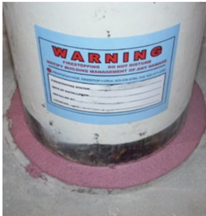
It is key that labels reflect the installed system. If not, it's a variance to the system and possible rejection. Performance Firestop Photo.
