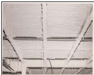
A Great Finished Deck
