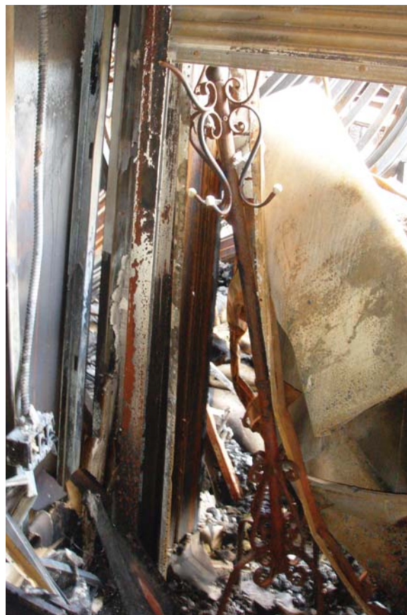
The closing path of rolling fire doors are required to be free of any objects that may interfere with door closing. Routine testing draws awareness to fire door locations and the need to keep their closing paths clear.
