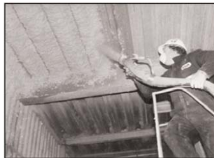
Applying the Proper Thickness
