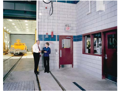
Fire Doors protect operations from offices importance to life safety.
