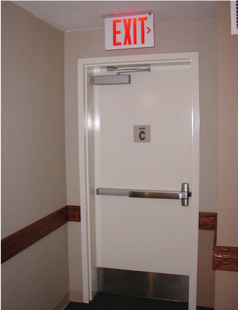
Fire resistance-rated doors, hardware and frames protect compartmentation continuity. Photo courtesy of Ingersoll Rand Security Technologies
