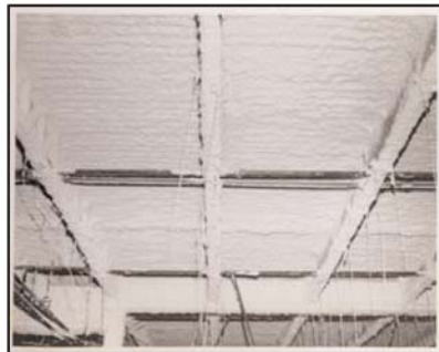
A Great Finished Deck
