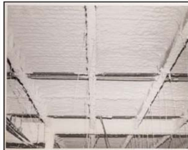
A Great Finished Deck
