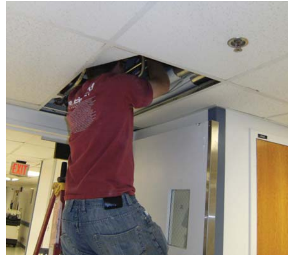
Working above ceilings requires care. (Photo courtesy of Multicon)
