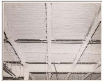
A Great Finished Deck
