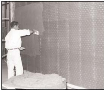
Fire Rated Walls
