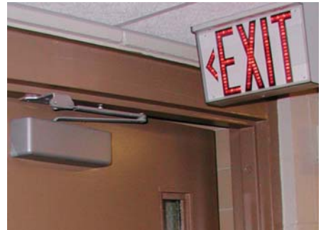
Door closers protect people and assets, as well as the door itself.
