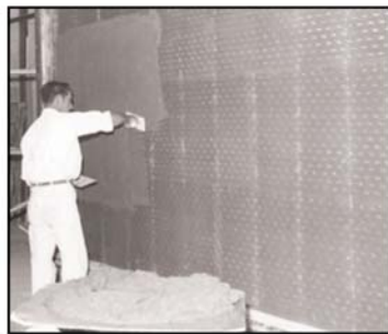
Fire Rated Walls
