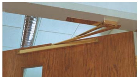
Overhead stop is visible with door open. Used here with concealed closer, it protects the door, hinges and closer from abuse or misuse.
