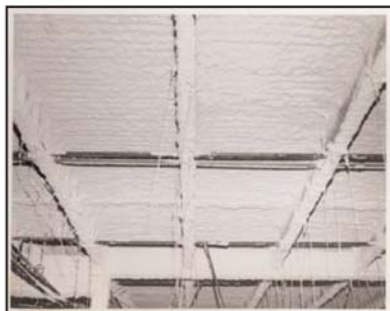
A Great Finished Deck
