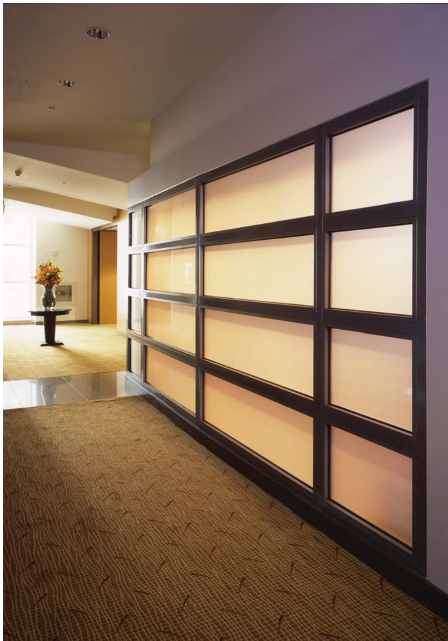
Pilkington Pyrostop glazing is fire-rated for up to two hours.
