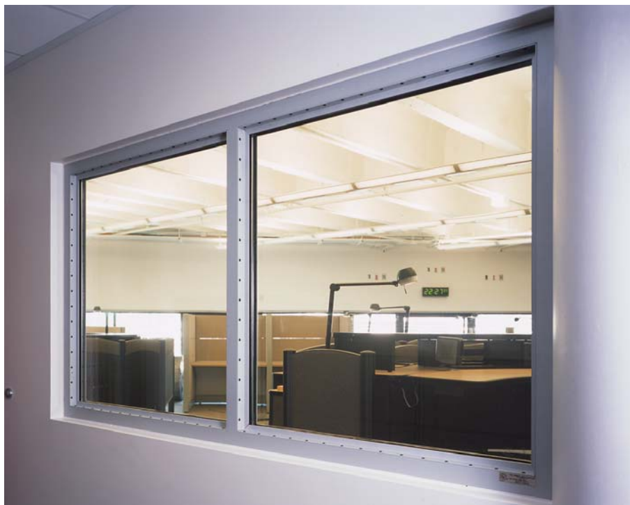
The Eastside 911 Communications Center in the Bellevue, Wash. City Hall uses Pilkington Pyrostop glass and FireFrames Heat Barrier frames.
