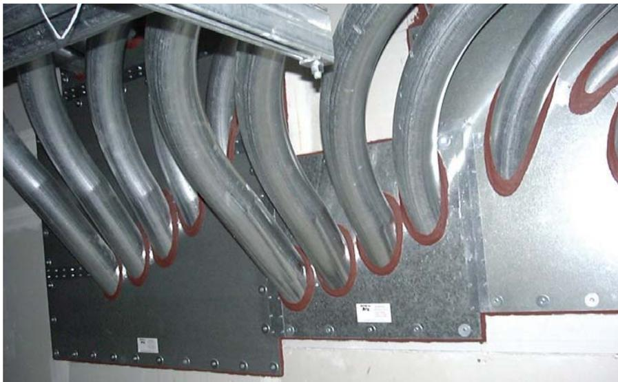
Compartmentation is completed when holes for conduits are sealed effectively to maintain the fire resistance rating of the wall. (Photos courtesy of Specialty Firestop Systems, Inc.)
