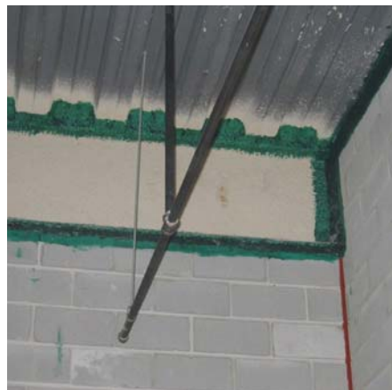
Compartmented walls are sealed for continuity around fireproofed beam. (Photo courtesy of NexLevel Construction Solutions Inc.)
