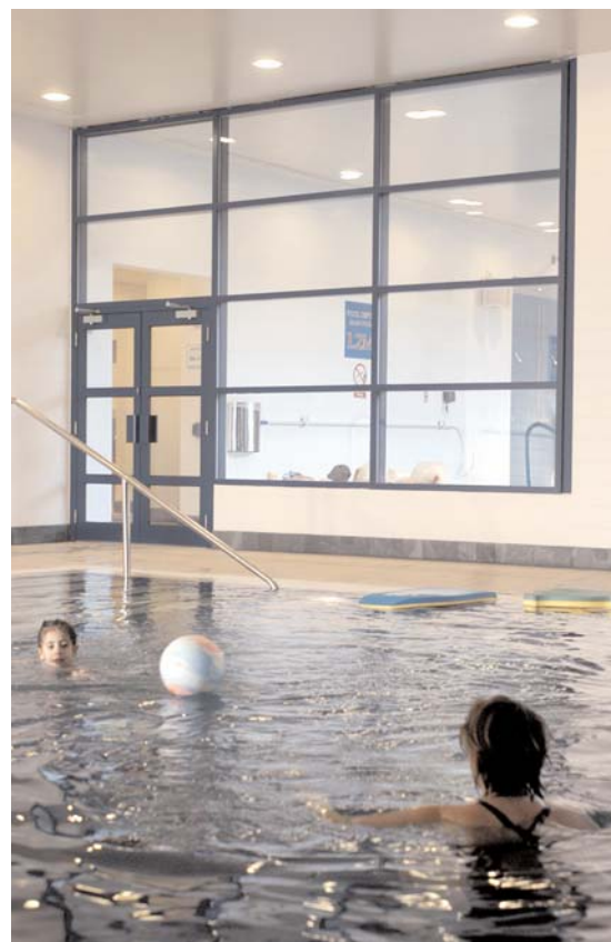
Fire protection glass barrier in concrete block at Holmes Place, Manchester, England. (Photo courtesy of Pilkington)
