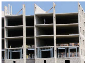
Precast concrete and masonry are often selected to satisfy minimum code requirements and provide superior construction, offering durable, safer and comfortable housing. (Photos courtesy of the Portland Cement Association)
