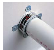
Firestopping installed to contractors' quality process results in a "system."
