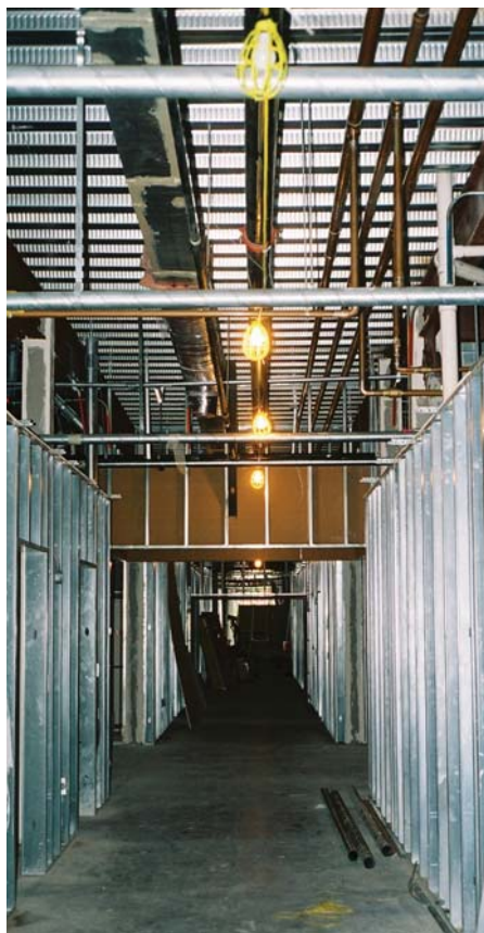
Construction and manufacturing environment differences are clear in this photo. (Photo courtesy of Specialty Firestop Systems Inc.)
