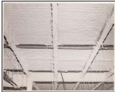
A Great Finished Deck
