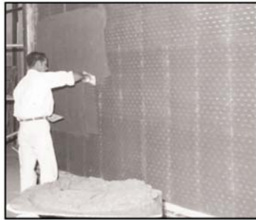
Fire Rated Walls
