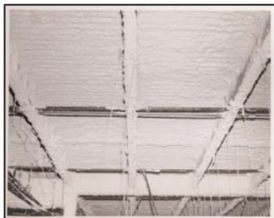
A Great Finished Deck
