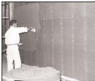
Fire Rated Walls
