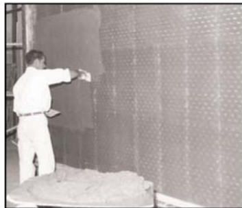
Fire Rated Walls
