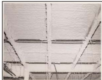
A Great Finished Deck
