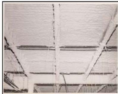
A Great Finished Deck
