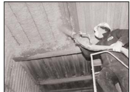
Applying the Proper Thickness
