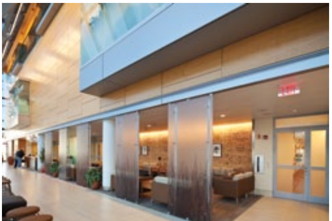
Lightly sandblasted full-lite fire-rated glass doors balance privacy with vision and blend in with the hospital's soothing design plan. TGP Photo
