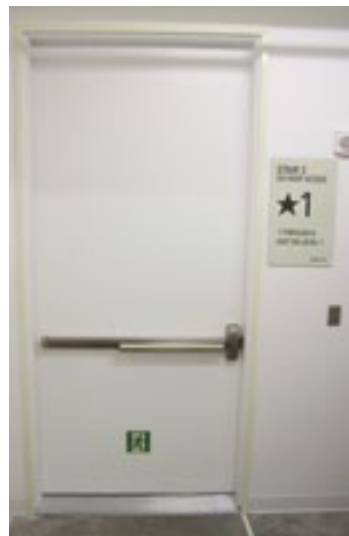
Top and sides of door frames, push bar + sign exit doors. American Permalite Photo
