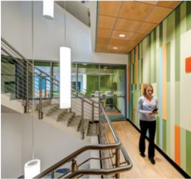
In Cincinnati Children's Medical Center, fire-rated glass and framing within a stairwell extends line of sight for occupants. TGP Photo
