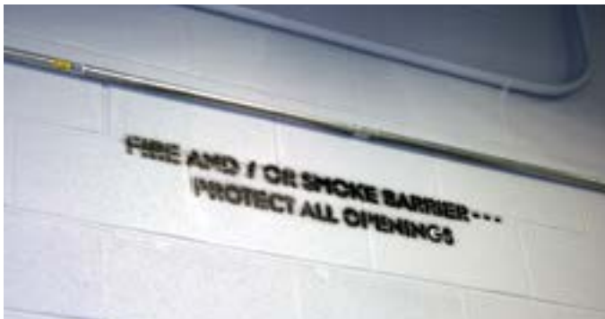
Fire-Resistance-Rated walls are required to be marked by the International Building Code. Heckler photo
