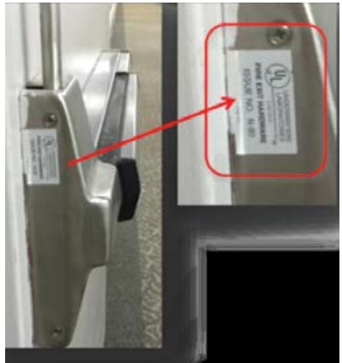
Door Hardware Label. Door Security Safety Foundation photo
