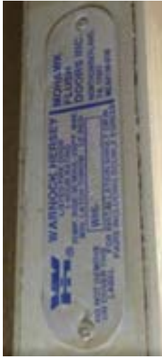
Fire Door marking - labels, with a lot of info, including hourly ratings. Door Security SafetyFoundation photo
