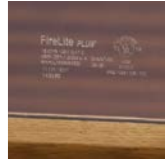
Fire-Rated Glazing has code requirements for labeling. TGP photo
