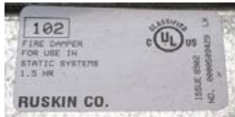
Fire Dampers have labels. Ruskin photo
