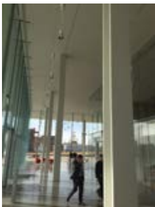
IFRM exposed in Lobby Carboline, K Building Specialties Photo
