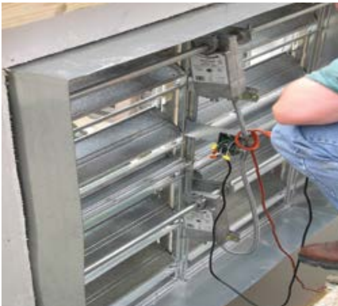
Fire Dampers get tested at installation, commissioning, 1st year, then in hospitals every 6 years, and other occupancies every 4 years. Ruskin Photo
