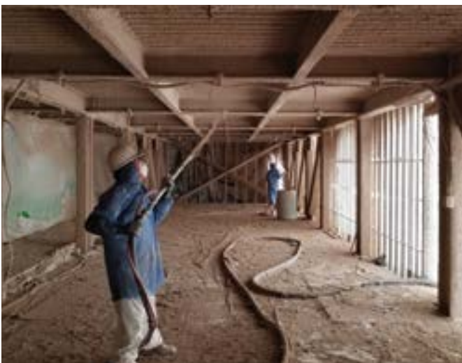
Spray fire resistive materials. Wohl Photo
