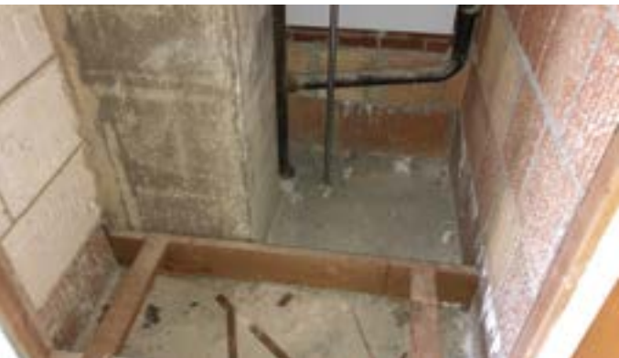
Gypsum block and clay tile wall assemblies have fire-resistance- ratings. C. Zussman, Pepper Constr. Photo
