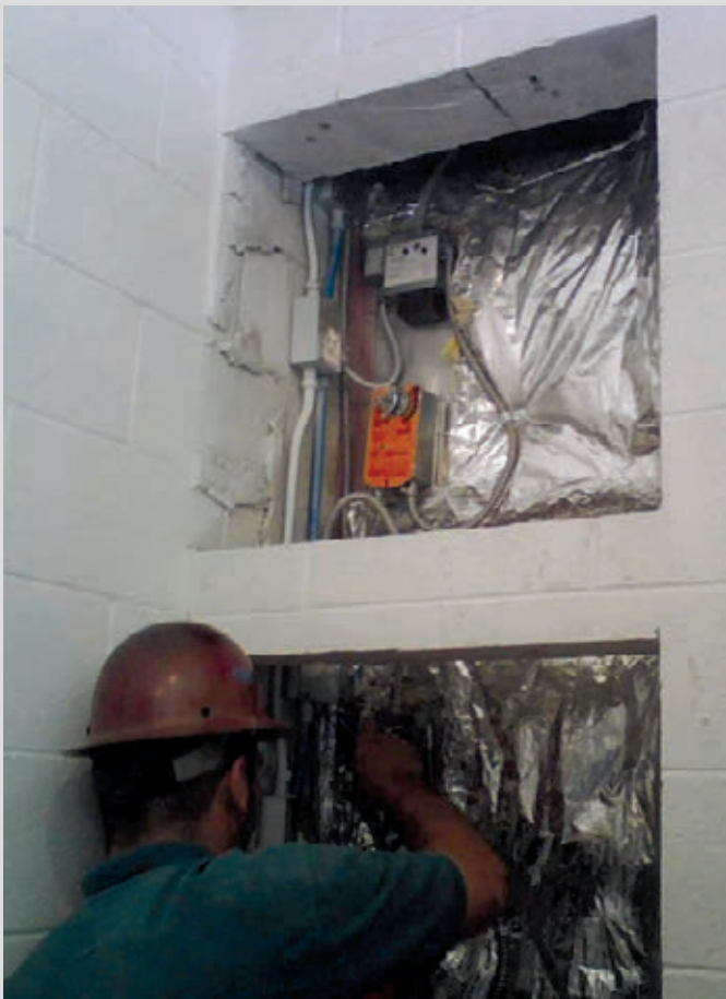
Fire Dampers are serviced by professionals who understand the dampers. Greenheck Photo
