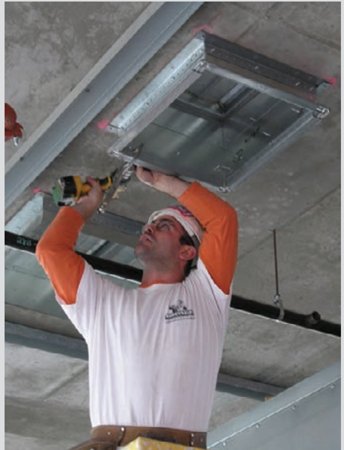
Fire Damper Angles protect the annular space around the damper, allowing movement. Greenheck Photo
