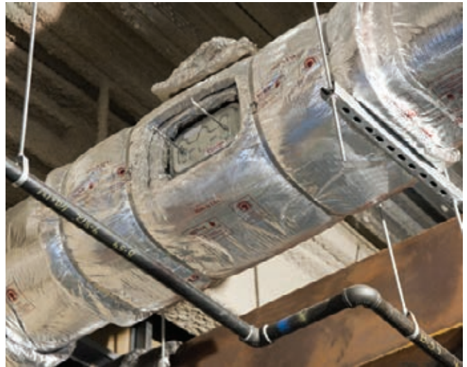
Fire resistance rated duct wrap layered prior to door application. Ductmate Photo
