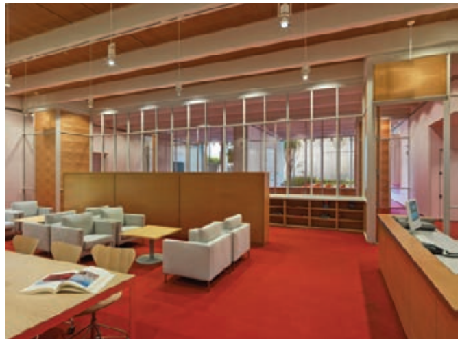
Tested to ASTM E119 standards, fire-rated transparent wall panels can be used for glass walls and partitions. Photo courtesy of Technical Glass Products
