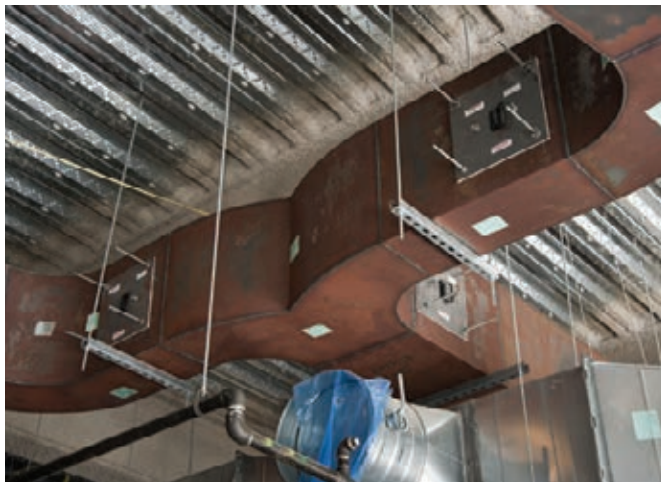
Bare grease duct prior to fire resistance rated ductwrap application. Note prefabricated doors with extra long threaded rods already welded in place. Ductmate Photo
