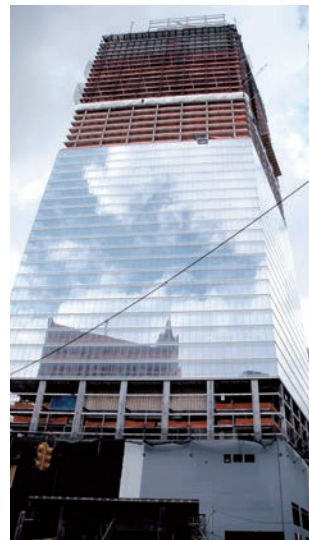
Steel frame High Rise Building. Grace Photo.
