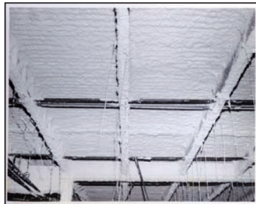
A Great Finished Deck
