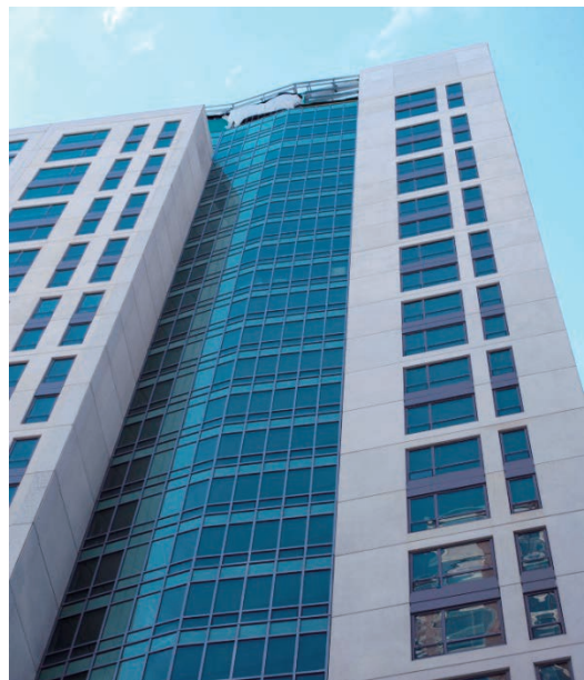
Part of The Kensington's west facing elevation featured a 1-hour curtain wall that integrated seamlessly. SAFTIFIRST Photo.
