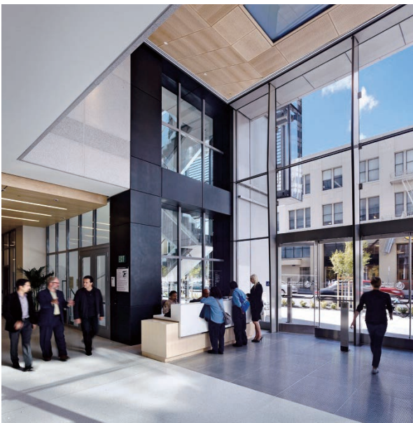
The 2-hour transparent stairwell, used in all 14 floors of the SFPUC, is situated prominently near the main lobby. SAFTIFIRST Photo.
