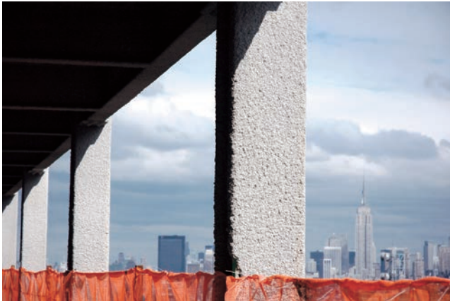
New York skyline with SFRM on steel columns. Photo of Grace Monokote MK-10HB. Grace Photo.
