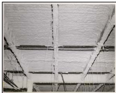
A Great Finished Deck
