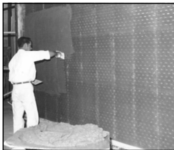
Fire Rated Walls
