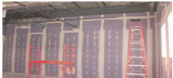
Fire-resistance rated walls must be installed to the tested system limitations to function as intended. FCIA Photo
