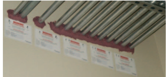
Firestop systems can be identified through labels. This sets up easier verification of the system during the maintenance of the building. PPMI Photo.
