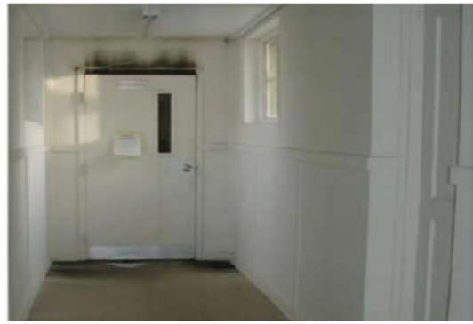
Swinging fire doors with rated builders hardware and rated frames installed to the tested system protect occupants. DHI Photo
