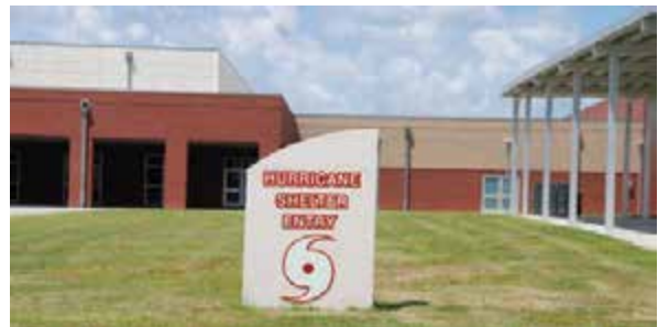
Figure 3: Hurricane/tornado shelter at West Harrison High School, Gulfport, MS. Source: Photo by Tim Burkitt / FEMA photo. FEMA.gov, visited 2013.
