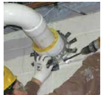
Trained installers get firestopping done right. Hamilton-Benchmark photo
