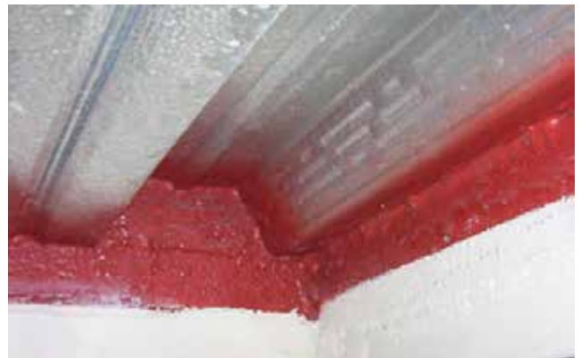
Firestop Spray installed to the listed system detail becomes a 'Firestop System'. Firestop Solutions, Inc. photo
