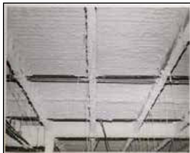
A Great Finished Deck
