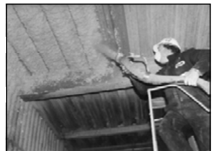
Applying the Proper Thickness
