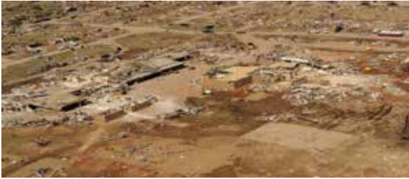
Figure 4: Plaza Tower Elementary School, Moore, OK, May 22, 2013. Source: FEMA.gov, visited 2013, Jocelyn Augustino/FEMA
