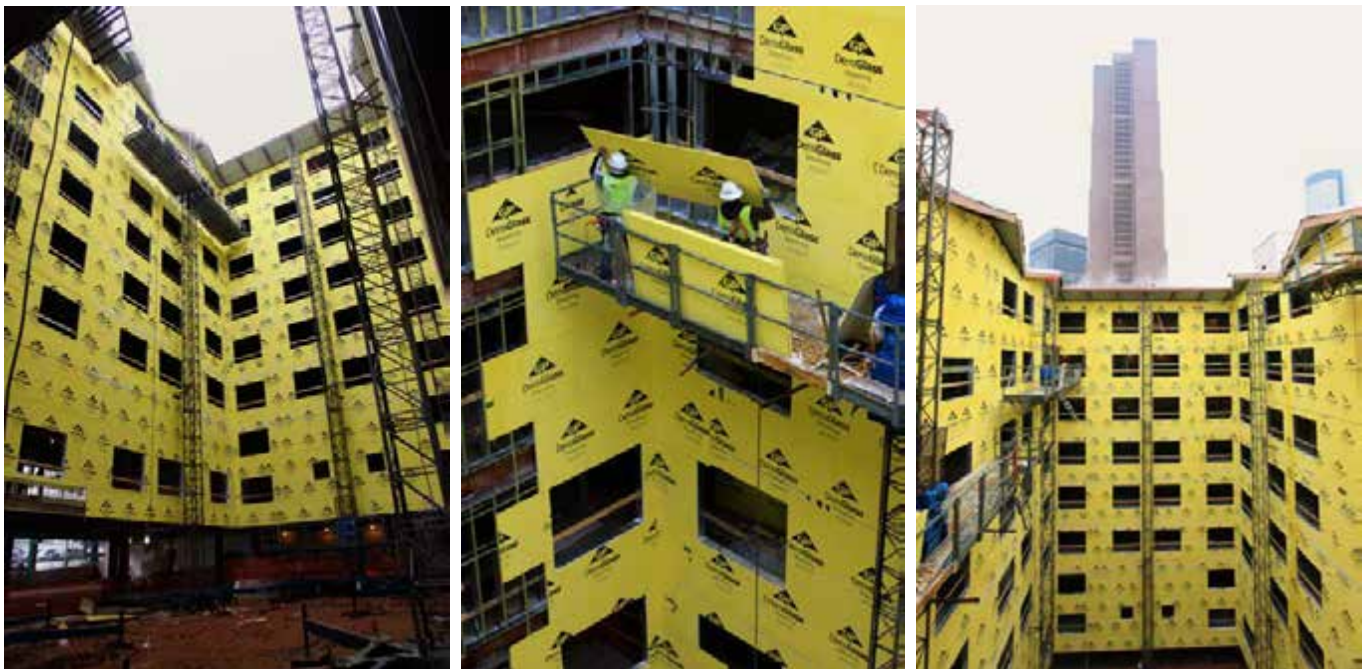
Fiberglass mat-based gypsum sheathing panels, like these Georgia-Pacific Gypsum DensGlass® panels installed on a student apartment complex in Atlanta, have excellent fire-resistant properties as part of a fire-rated exterior wall assembly. The exterior wall system, part of the building envelope, provides structural support; air and water resistant barriers; insulation and an attractive cladding for a beautiful building built to last.
