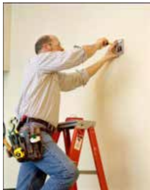
A speaker strobe being installed
