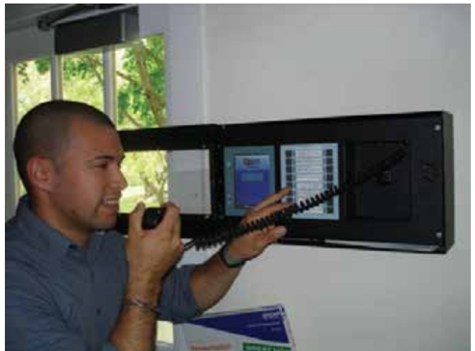
A Local Operator Console from Gamewell-FCI enables authorized users to send live voice alerts or pre-recorded messages through the fire alarm/emergency communication system
