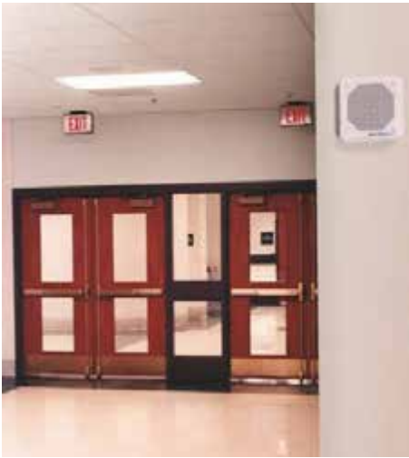
ExitPoint Directional Sounder from System Sensor positioned by a school building's main entryway and exit
