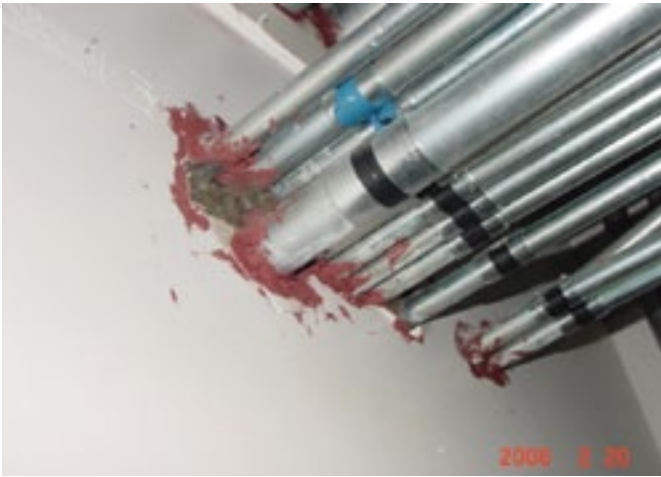
NFPA 1 states that improper installation is the building owner's responsibility. Specialty Firestop Services Photo.
