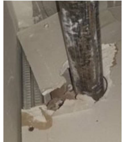
Breaches made for penetrating items. Some are not pretty. Pro-Firestop Photo
