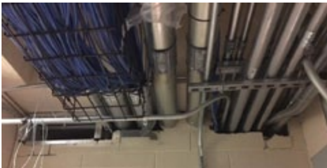
Open breaches happen. Pro-Firestop Photo
