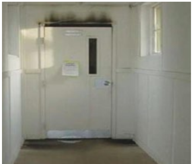
Fire doors keep areas safe. Door Security & Safety Foundation of the DHI Photo
