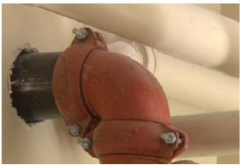
Breaches made in barriers for piping, electrical and other penetrations need protection. TJC Photo
