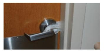
Fire Doors are supposed to close and latch to be effective. Hold open devices are not allowed. TJC Photo
