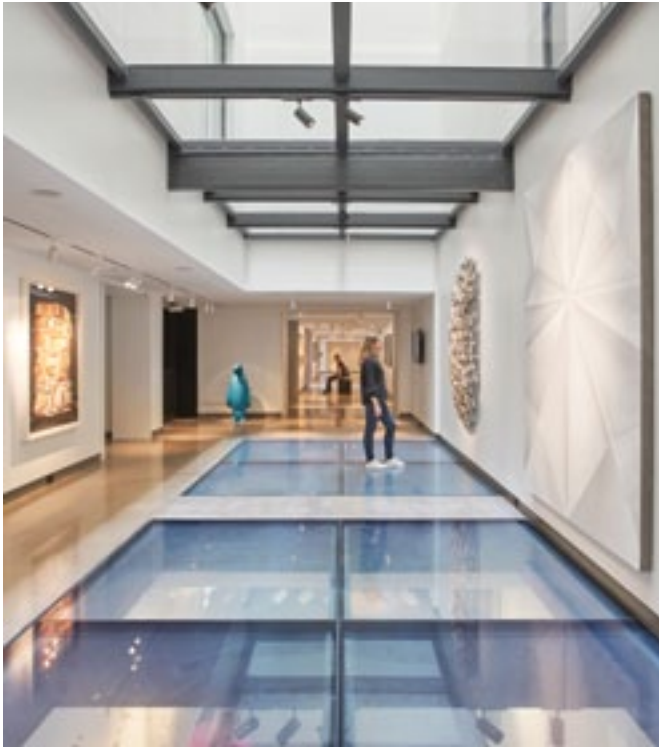
Fire-resistive glazing floors tested to ASTM E-119/UL 263 allows daylight to penetrate further into the building while meeting fire-resistance-rated requirements. SAFTI FIRST photo.
