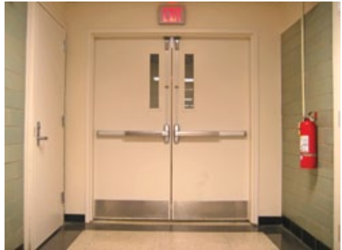
Fire Rated Cross Corridor Doors in High School. bobelias/Bigstockphoto.com Photo.
