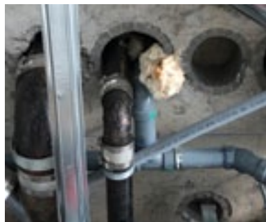
The grey penetrating item was added to the annular space where a cast iron penetrating item exists. Compliance without a collar? FCIA Photo
