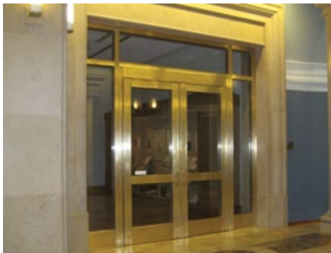
90-minute fire-resistance-rated temperature-rise pair doors with custom brass cladding at University of California at Berkeley Doe Library in Berkeley, CA. SAFTIFirst Photo.
