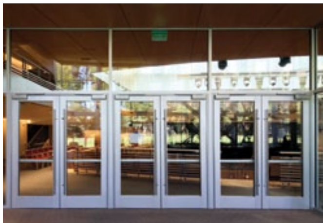
90-minute fire-resistance-rated temperature-rise pair doors with a clear anodized finish at Harvard Business School's Klarman Hall in Boston, MA. SAFTIFirst Photo.
