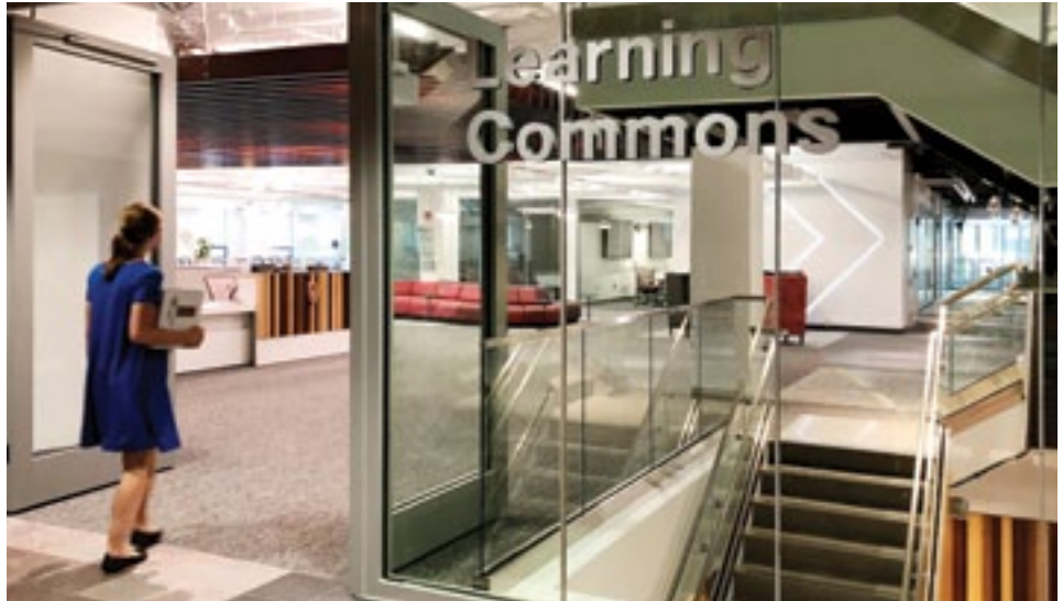
These 9-ft high 60-minute fire-resistance-rated temperature-rise pair doors matches the height of the adjacent 1-hour butt-glazed wall at the University of Wisconsin School of Business Learning Commons in Madison, WI. This eliminates the need to add a transom to the door assembly, which appealed to the architect. SAFTIFirst Photo.
