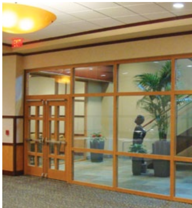
90-minute fire-resistance-rated temperature-rise pair doors with wood veneer finish at Reid Hospital in Richmond, VA. SAFTIFirst Photo.
