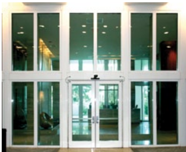
90-minute, fire-resistance-rated temperature-rise and hurricane-rated pair doors at the Las Olas Beach Club in Ft. Lauderdale, FL. SAFTIFirst Photo.
