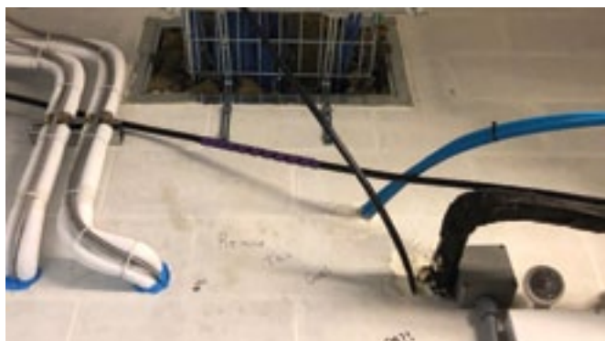
Single and multiple pipe cable penetrations treated might or might not be compliant. The documentation or 'Inventory' is needed to be sure. FCIA Photo
