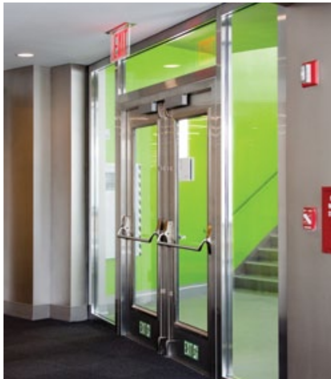
90-minute fire-resistance-rated temperature-rise pair doors with stainless steel finish at City University of New York (CUNY) School of Law in Long Island City, NY. SAFTIFirst Photo.
