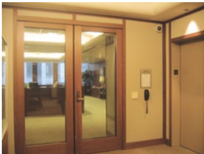
60-minute fire-resistance-rated temperature-rise and ballistic-rated pair doors for a private office in San Francisco, CA. SAFTIFirst Photo.
