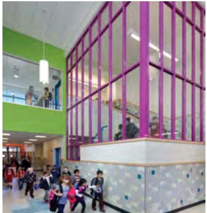
A brightly colored fire-resistance-rated curtain wall system reflects the playful energy of students. TGP Photo.
