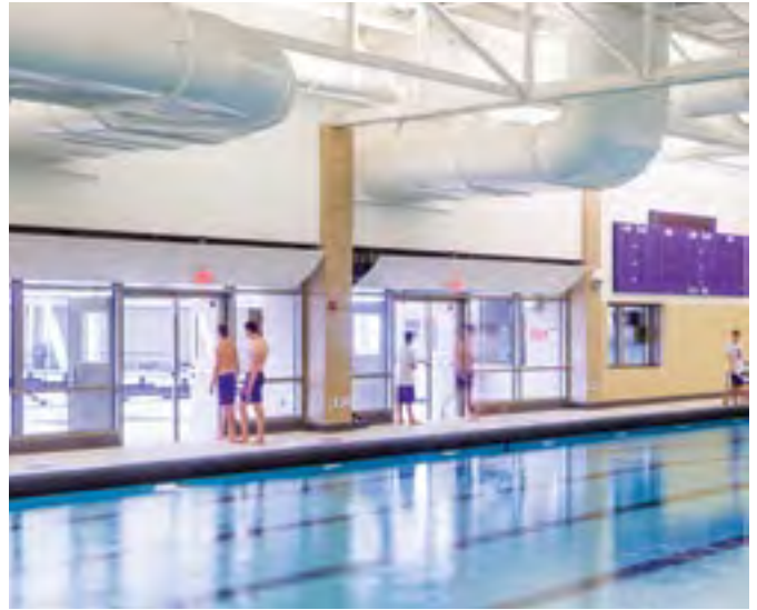
A two-hour fire-resistance-rated glazing separation enhances visibility in a high school aquatics center. TGP Photo.
