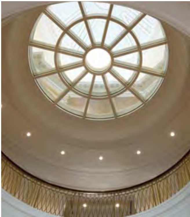
In CNU Student Success Center, a fire-rated glass system improves light transfer while providing critical fire resistance. Virginia Hamrick and Glavé & Holmes Photo.
