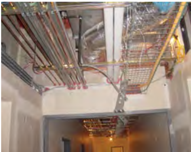
Specialty Firestop, Inc. photo
