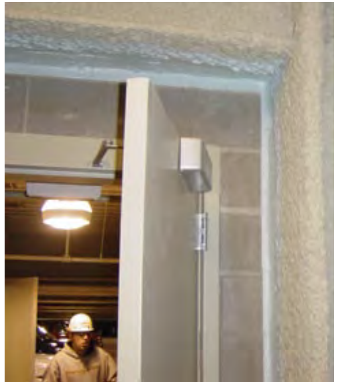
Specialty Firestop, Inc. photo
