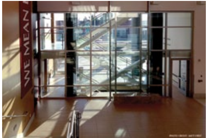
To meet code and provide transparency and natural light, fire-resistive glass and frames were used in this 2-hour stairwell application. Project: University of Utah David Eccles School of Business. Architect: MHTN. Glazier: Mollerup Glass. Products: SuperLite II-XL 120 (wall) and SuperLite II-XL 90 (door) in GPX Architectural Series Framing Photo: SAFTI FIRST
