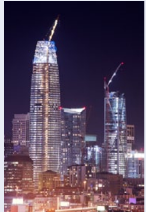
The Salesforce Tower in Construction Photo: Owens Corning
