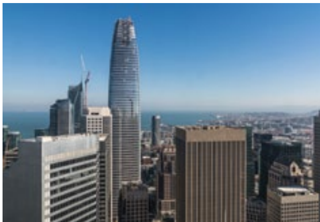
The curved exterior of the Salesforce Tower in San Francisco required a unique approach to perimeter fire-containment. Owens Corning/Thermafiber photo.
