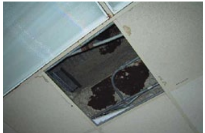
SFRM or IFRM can be damaged when new services are added to existing buildings and need repair and documentation of the repair to comply. GCP Applied Technologies Photo
