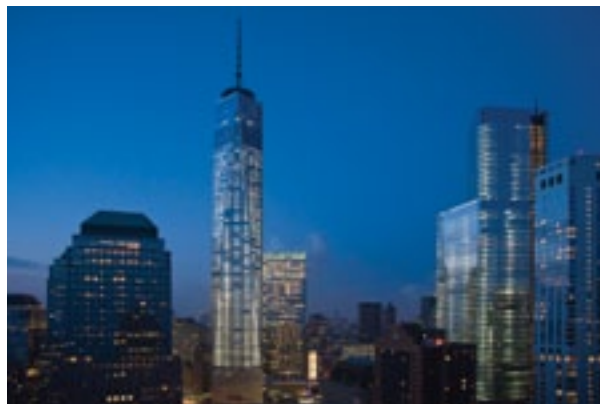
Four out of five of the tallest buildings in North America trust mineral wool. Owens Corning/Thermafiber photo.
