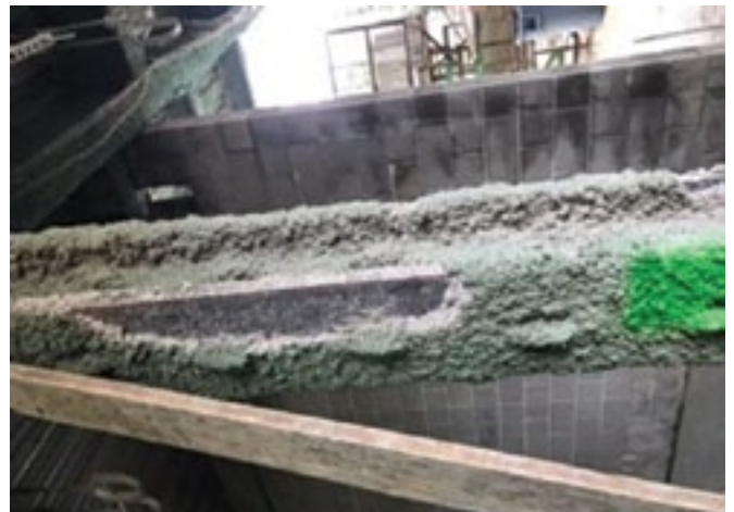
SFRM or IFRM can be damaged during construction, then repairs are needed. GCP Applied Technologies Photo
