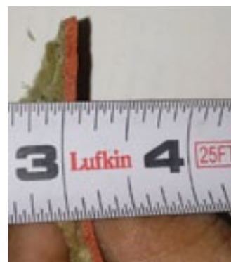
Firestop inspection equipment is not complex. Measuring tapes are used to determine thickness acceptability after calculating or sealant shrinkage. Firestop Southwest Photo.
