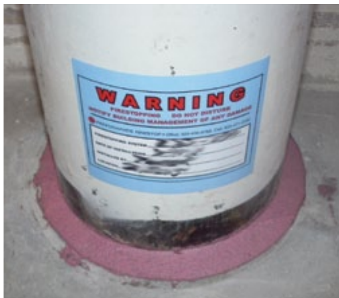
Firestop products become systems when installed to the listing and manufacturers installation instructions. Performance Firestop Photo.
