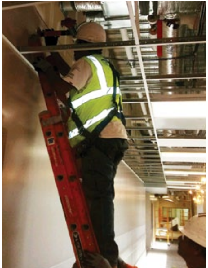
Firestop Inspection is many times above ceilings. Firestop Southwest Photo
