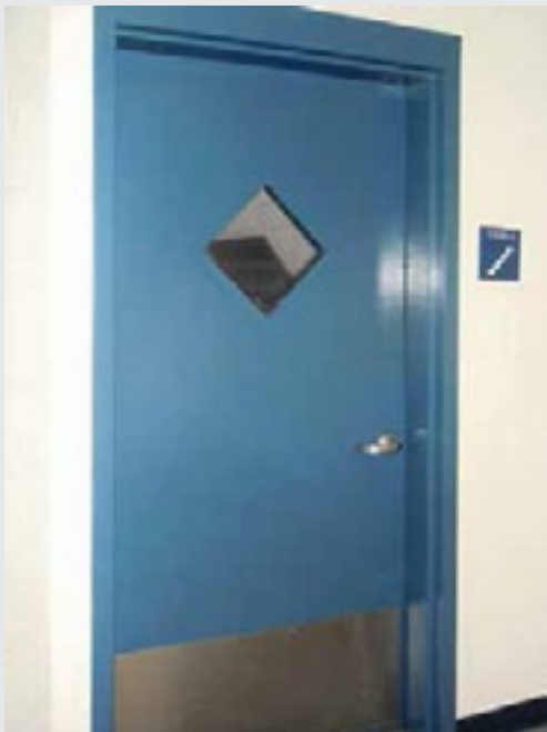
Filmed or Laminated Ceramic in a 60 minute temperature rise door limited to 100 square inches
