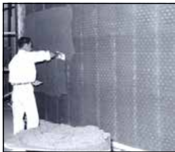
Fire Rated Walls
