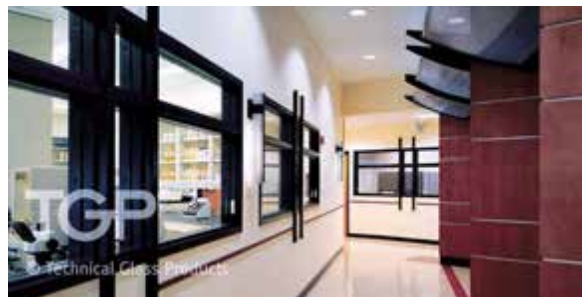
Fire rated glazing used to separate a laboratory from a corridor. TGP Photo
