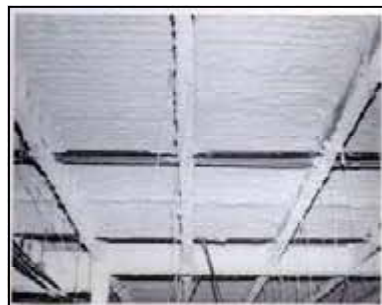
A Great Finished Deck
