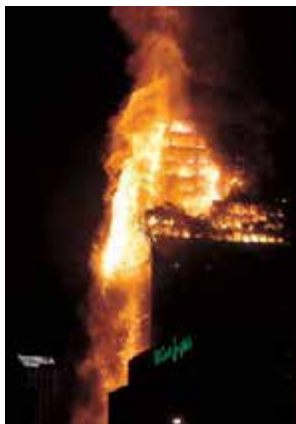
Windsor Tower Fire in Madrid, Spain. Juan Carlos Rohas, © Dusko Despotovic/Corbis
