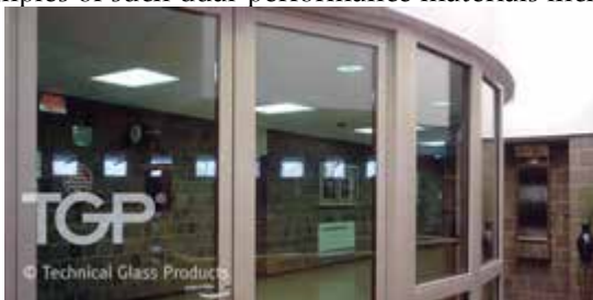
Fire rated glazing used as a separation for a corridor in a school. TGP Photo
