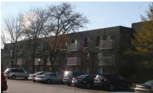
Terrace Apartments. Mansard roofs allowed fire to travel from balcony to open attic spaces. Keyworth photo.
