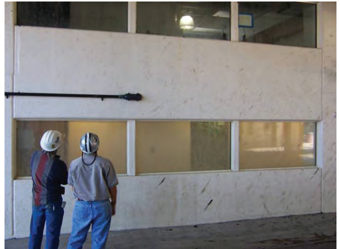
Fire rated glazing provides continuity of fire resistance and a view of important work areas. Pilkington photo.
