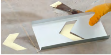
Epoxy Casting Resin (a paste, NOT a paint) that gets applied using a stencil and a spatula. American Permalite photo.
