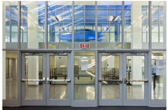
Fire rated glazing allows light into stairwells. Pilkington Photo.
