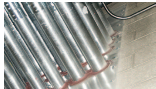
Specialty Firestop Contractors understand how to install firestop composite sheets to the systems documentation efficiently. PPMI photo
