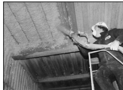
Applying the Proper Thickness
