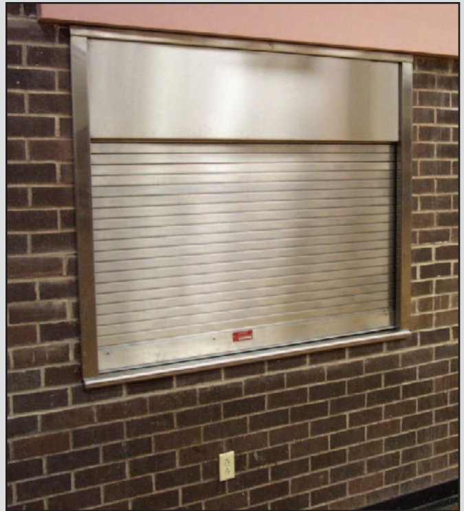
Rolling Fire Door in Masonry Construction. Cornell Photo
