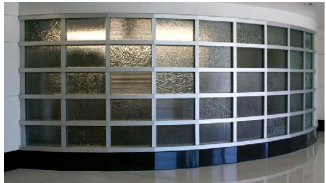
Fire Rated Glazing can be decorative. SAFTI Photo
