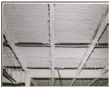
A Great Finished Deck
