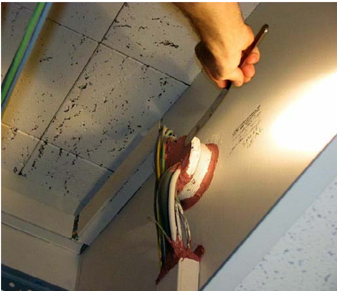
Firestop sealants are tooled. Gleeson Powers Photo
