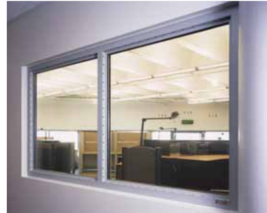
The Eastside 911 Communications Center in the Bellevue, Wash. City Hall uses Pilkington Pyrostop glass and FireFrames Heat Barrier frames."
