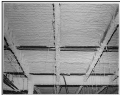
A Great Finished Deck
