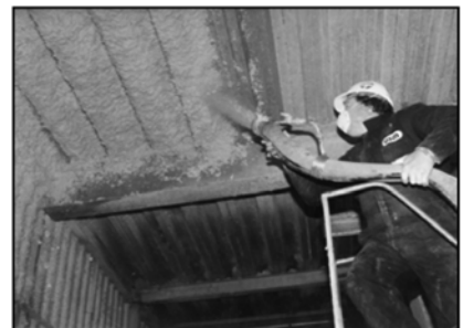
Applying the Proper Thickness
