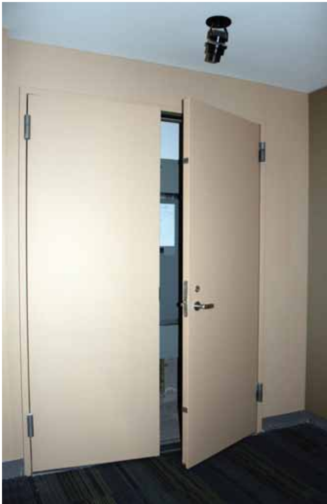
Large openings protected with fire doors
