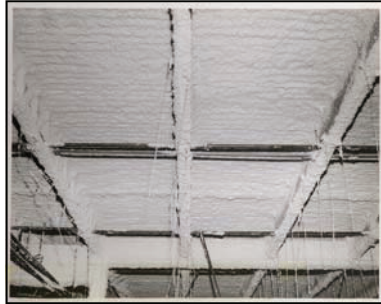
A Great Finished Deck
