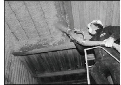
Applying the Proper Thickness
