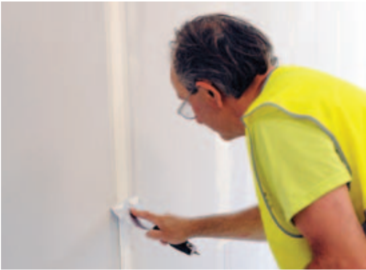
Joint taping for fire resistance continuity – LaFarge Photo
