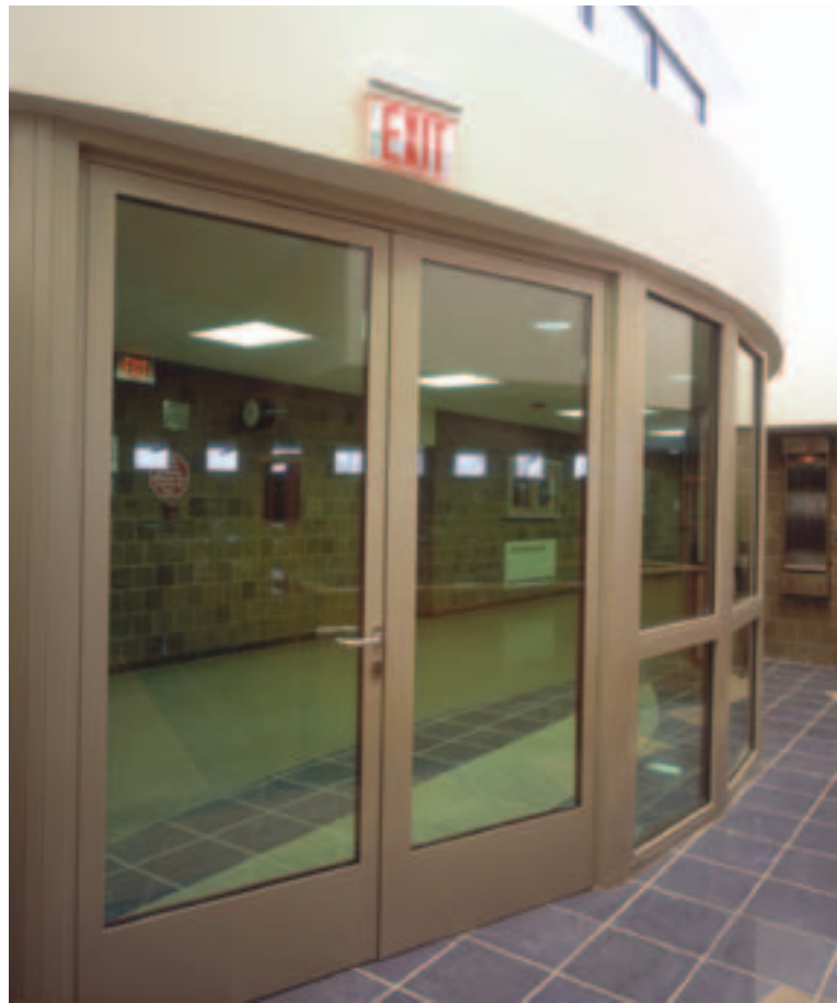
Fire rated glazing isolates corridors – TGP Photo
