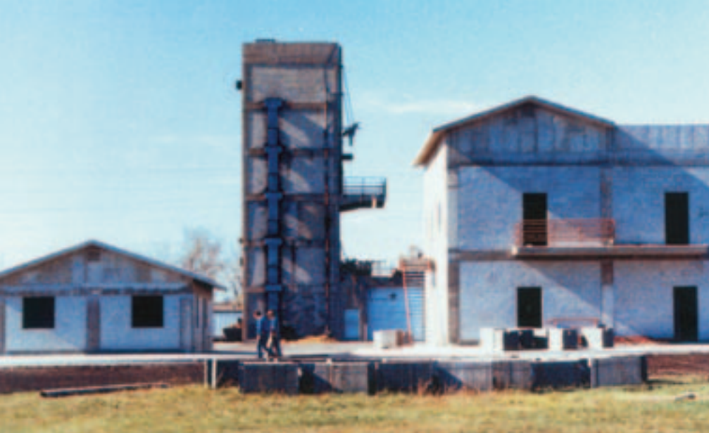
Fire resistance rated concrete training towers are used over and over again. — IL Masonry Institute Photo
