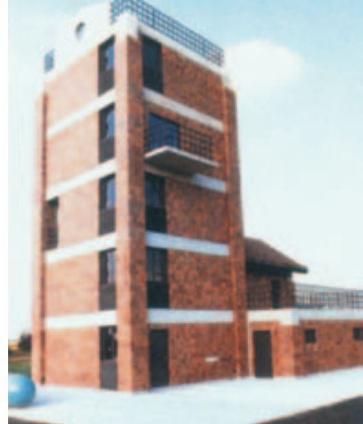
Concrete block walls and concrete floors provide environment for fire service training. — IL Masonry Institute Photo
