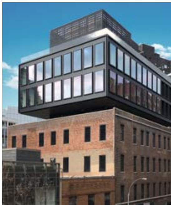
The 2-hour fire-resistance-rated exterior glass walls at The Warehouse on 520 W 20th Street have the largest tested and listed individual panel sizes for fire-resistance-rated glazing in the USA. SAFTI FIRST photo.
