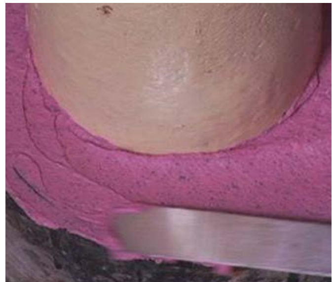
Firestop sealants are all required to be smoothed in the manufacturers installation instructions. The C-AJ-1353 will not mention this detail. That's why both the UL or other system, the manufacturers installation instructions and safety data sheets are needed for correct installation. FCIA Photo
