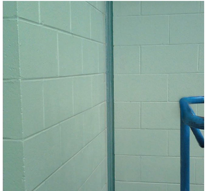
Vertical installation of a single-unit fire-rated expansion joint installed in a wall. UL-certification applies to walls constructed of fire-rated concrete, concrete blocks or gypsum. EMSEAL Photo
