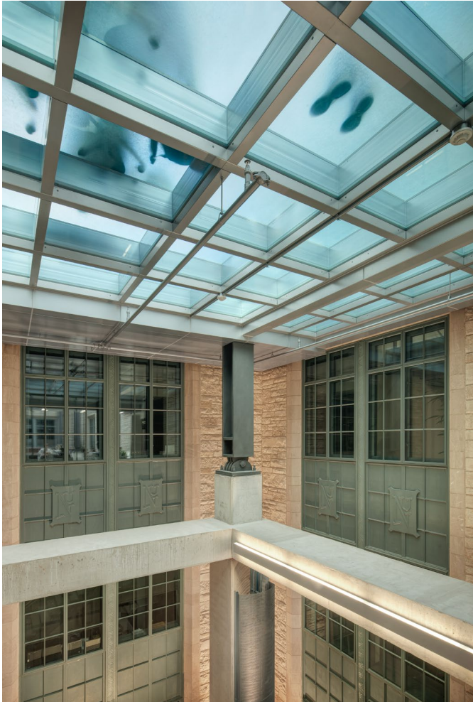
A fire-resistance-rated glass floor system provides compartmentation without restricting daylight to the floors below. Photo courtesy of TGP.
