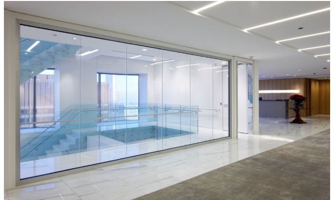
Design professionals can use butt-glazed fire-resistance-rated glazing system in areas where the building code requires fire-resistance and uninterrupted views are desirable. Photo courtesy of TGP.
