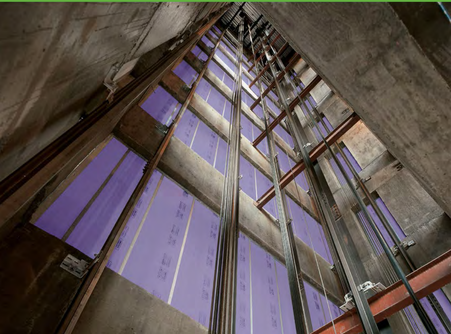
Interior view of elevator Cavity Shaftwall System utilizing PURPLE® shaftliner. Photo courtesy of National Gypsum Company.
