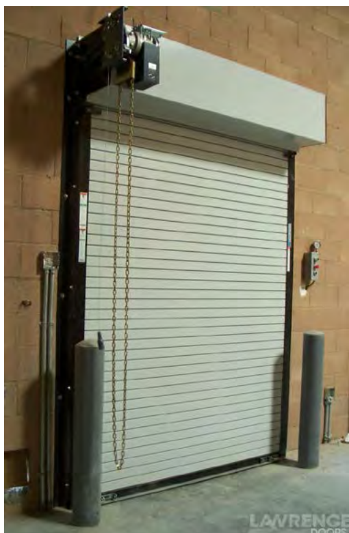
Insulated fire door installed on opening in outside wall
