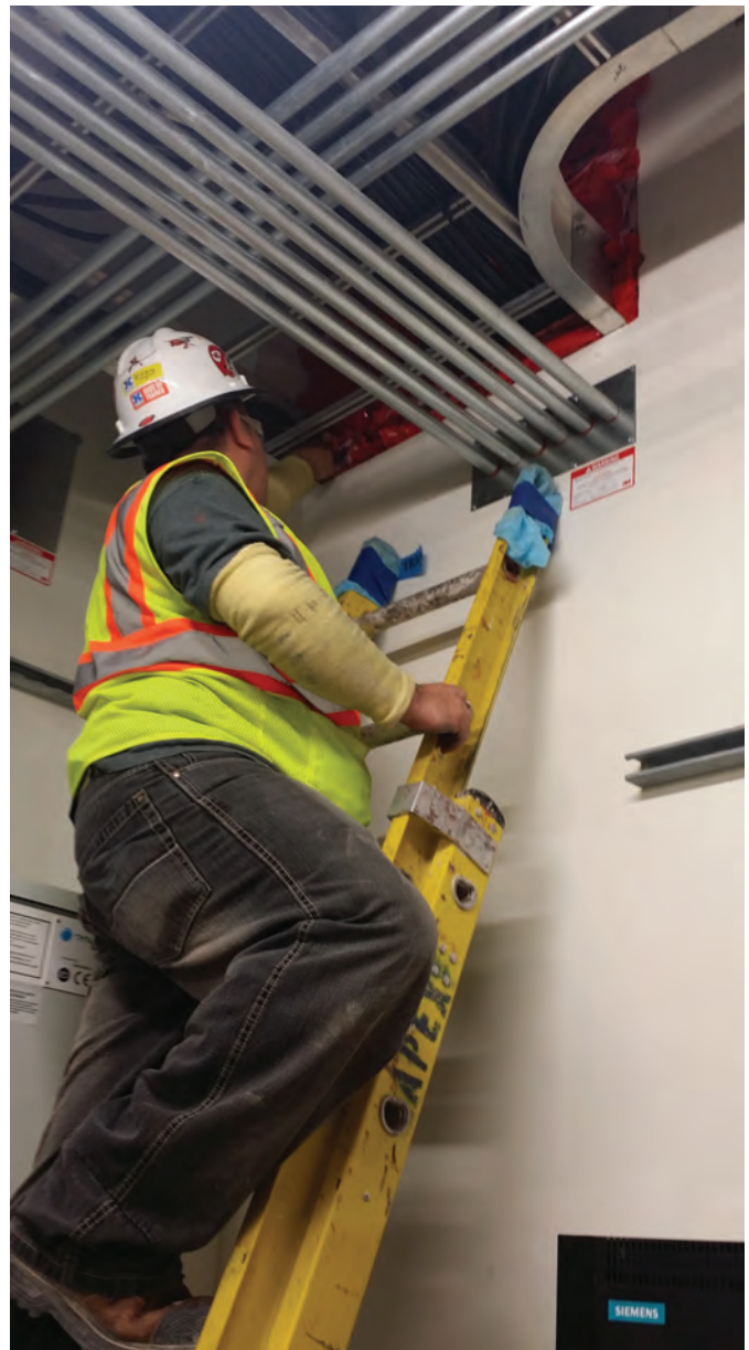
Figure 2: FCIA Photo, Apex Firestopping
