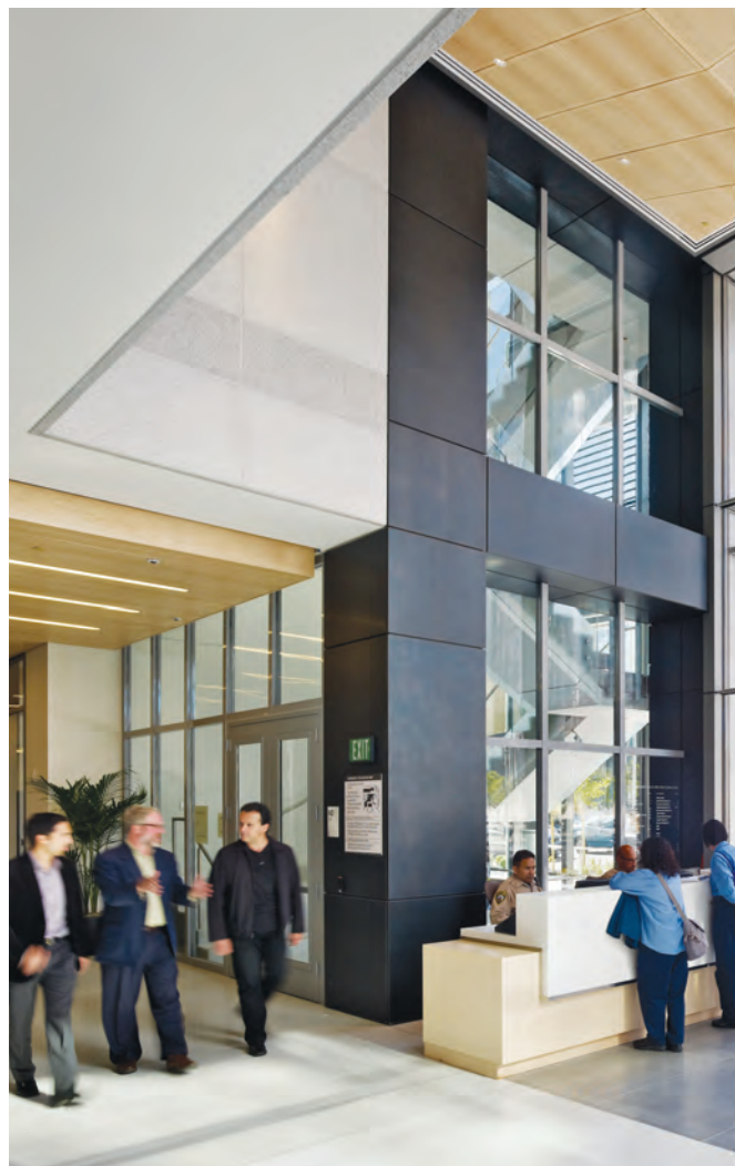
SuperLite II-XL 120 in GPX Framing is used on all 14-floors of the LEED Platinum-certified San Francisco Public Utilities Commission Building. SAFTIFIRST Photo
