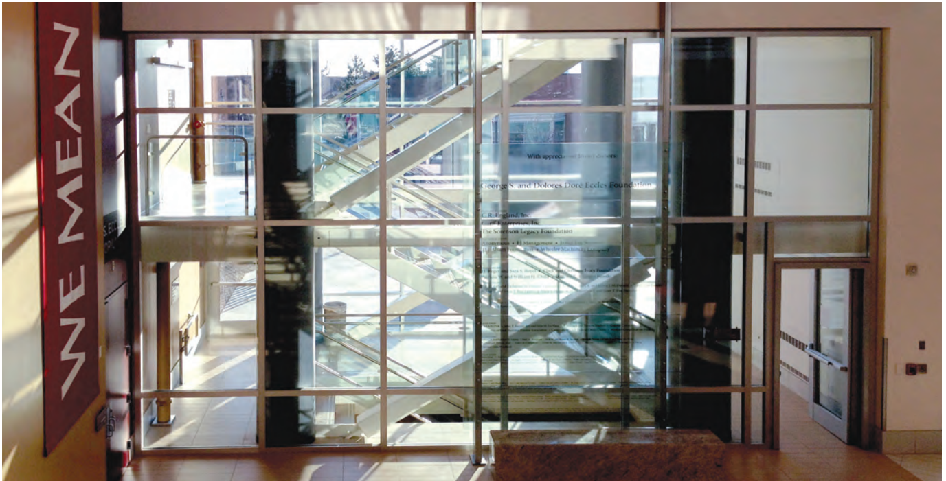
SuperLite II-XL 120 in GPX Framing add daylight and transparency to this 2-hour stairwell. SAFTIFIRST Photo
